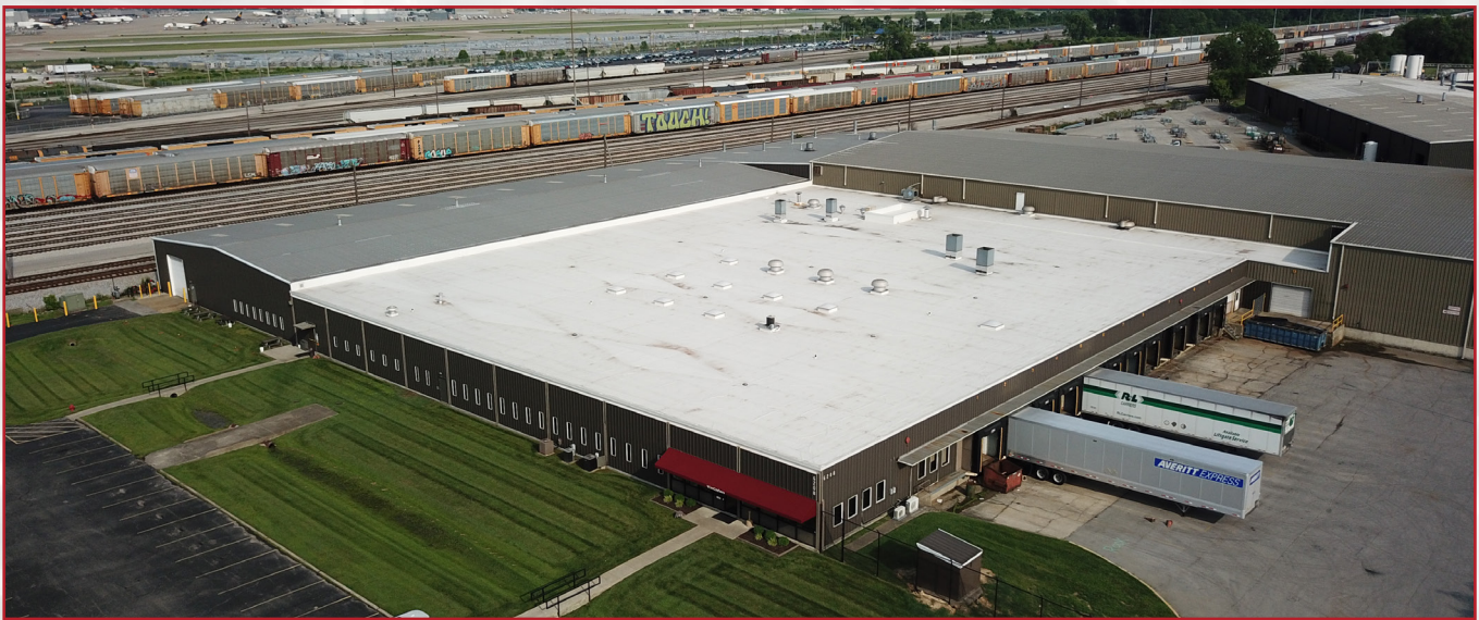
Aerial view of the WireCrafters facility.
